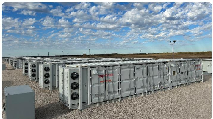
Rated Energy of LFP Battery: 71MW/129MWh
