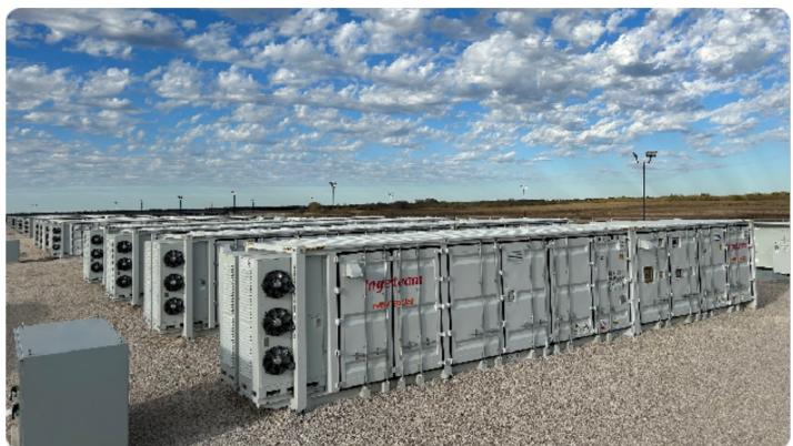
Rated Energy of LFP Battery: 71MW/129MWh
